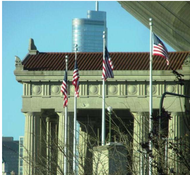
Clay Tile Roof installed by Mortenson Roofing, Soldier Field, Chicago, IL
