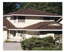
125 miles per hour that would strip off most other roofing materials. Testing has also shown concrete tile roofing systems, when installed according to building code standards, exceed current seismic load requirements for building materials.
