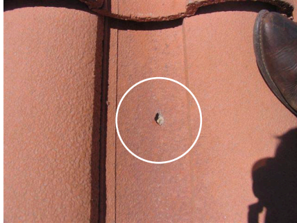
Pictures of chipping to edge of slurry-coated tile
