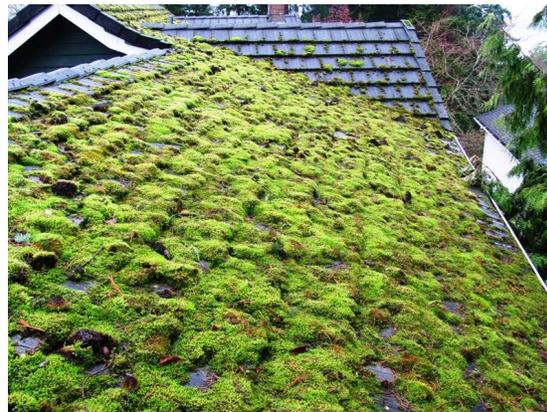
An extreme example of unchecked moss and tree debris on a 30-yr roof in a cool humid climate.
